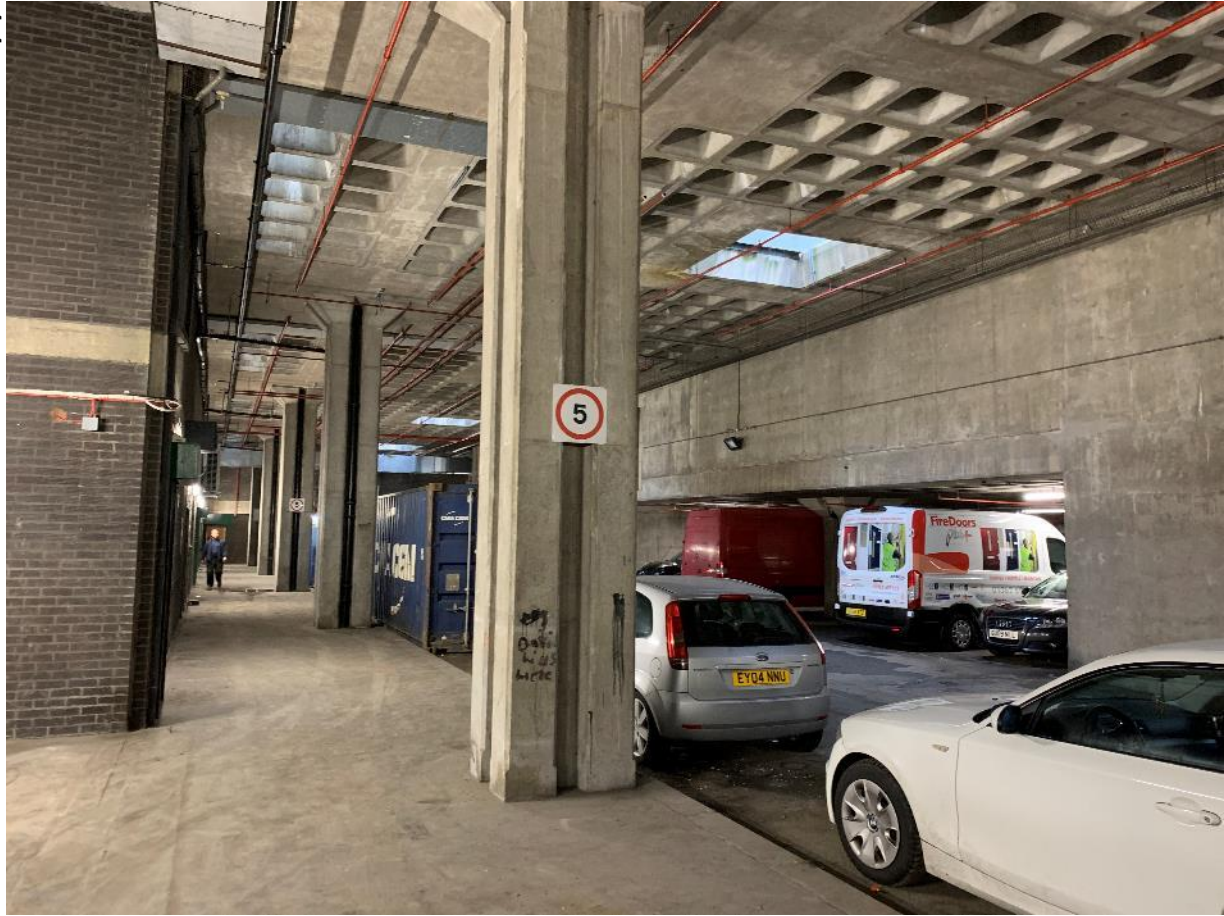
Looking towards Gravel Lane ↑
