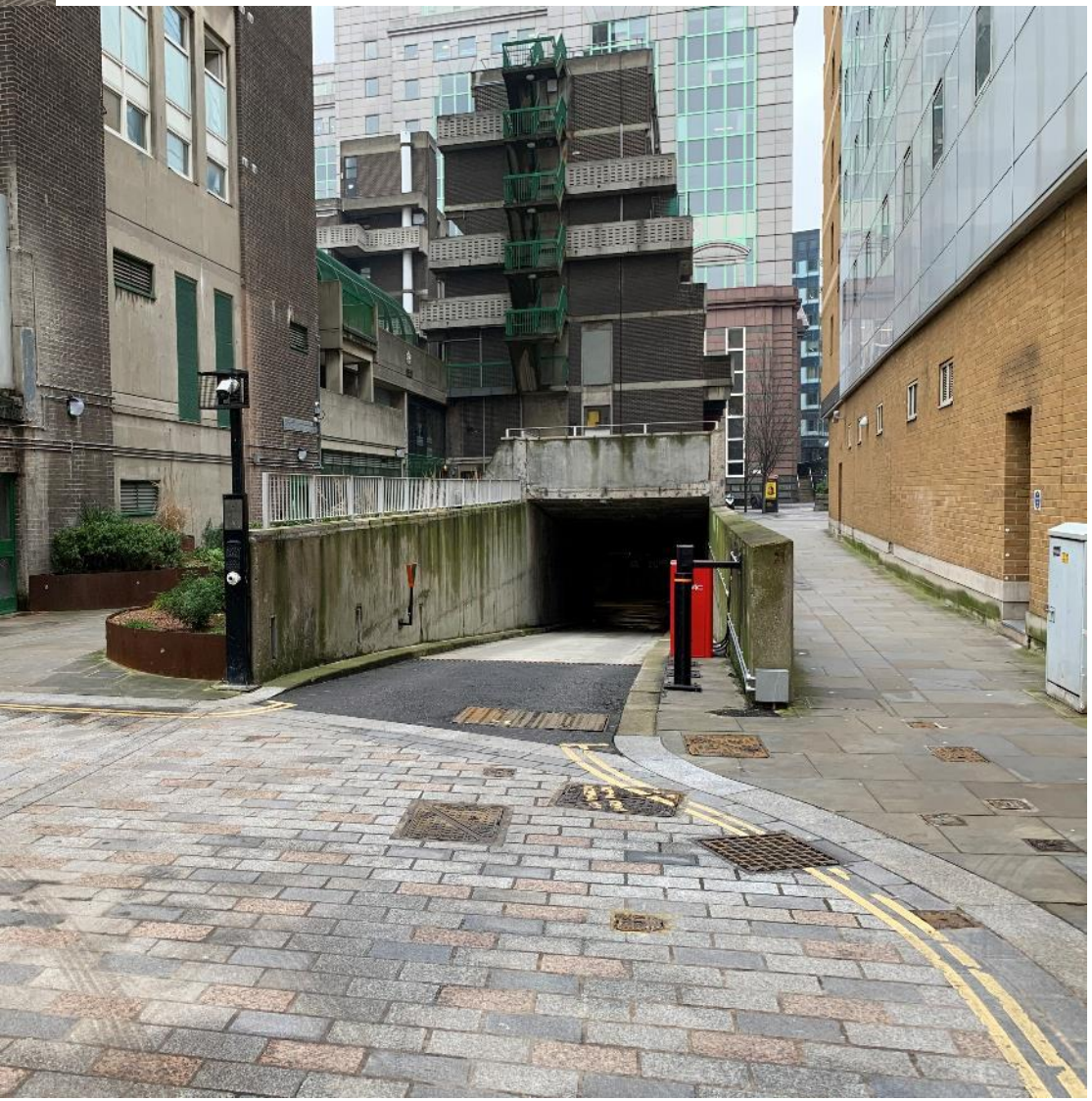
↑ Ramp to Basement Parking
